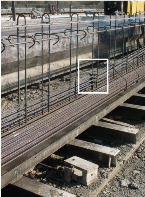
Figure 3.9 Typical Deflected Strands at Precast Plant C
