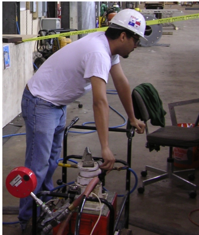
Figure 4.7 Load Being Applied by Pump
