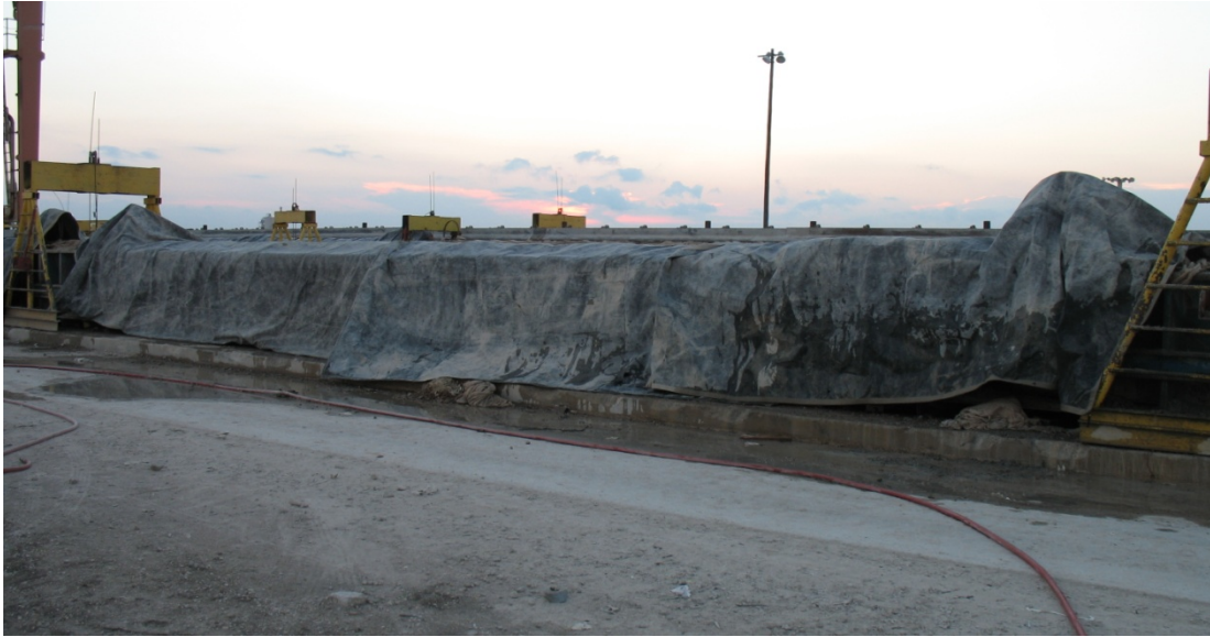
Figure 3.11 Typical Tarp on Beam during Curing Process
